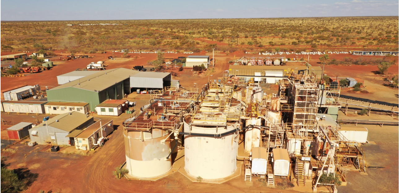
Figure 3: Coyote 300,000tpa processing facility which could be expanded to 700,000tpa with Black Cat's spare ball mill located in Kalgoorlie
