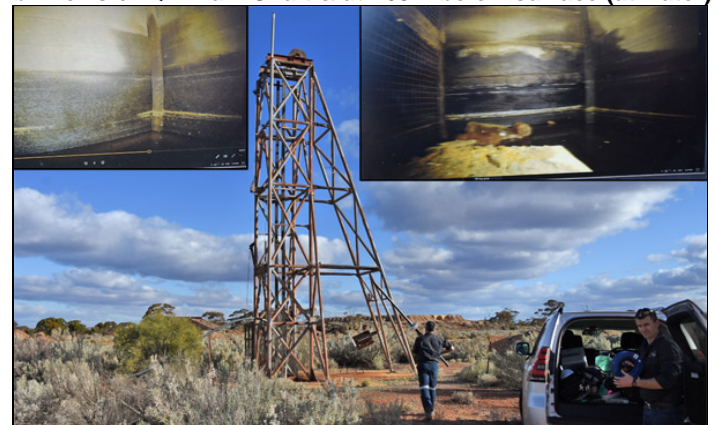
b. Views of QM Main Shaft & at ~65m below surface (at water)
