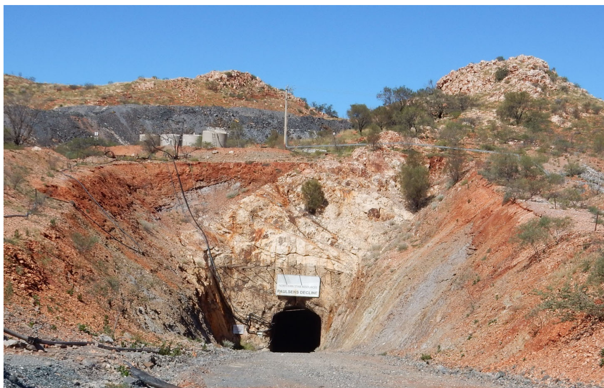
Figure 1: Paulsens underground mine is dewatered and ventilated with underground drilling planned for 2022
