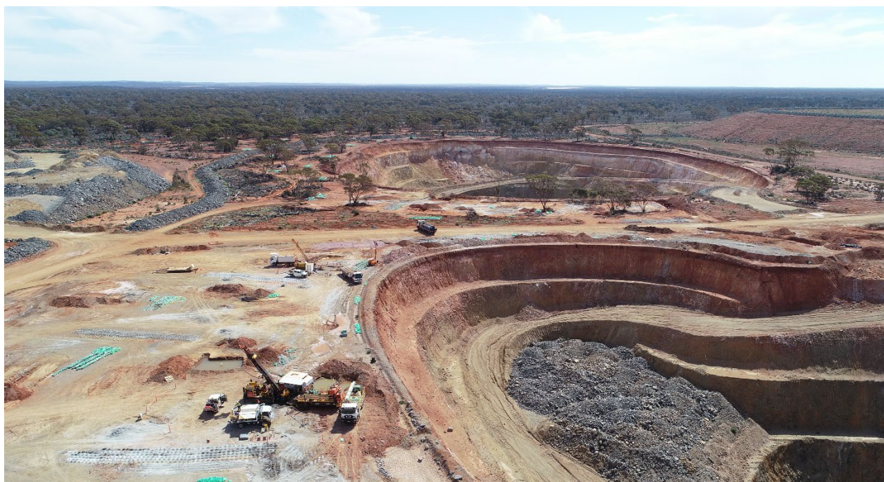
Figure 1: Multiple rigs at the Majestic mine site
