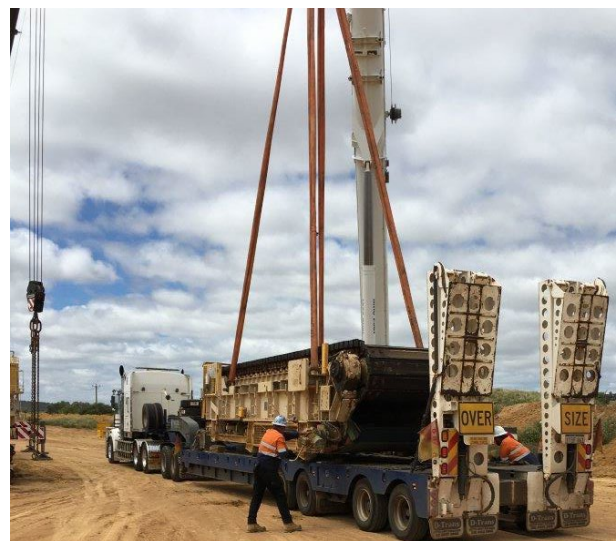
Figure 9: Apron feeder relocation to site during October 2021
