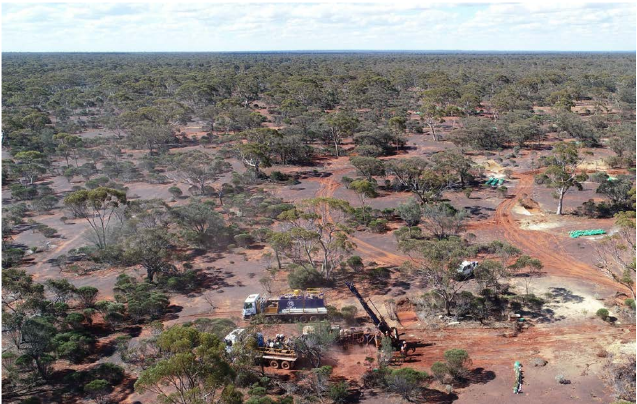
Figure 2: RC rig drilling at the Boundary Deposit, Bulong.
