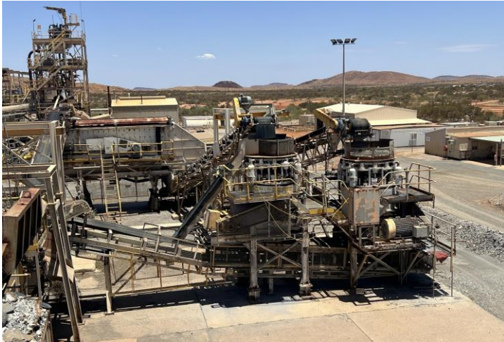
Crushing circuit: 100tph – proof run (operational)
