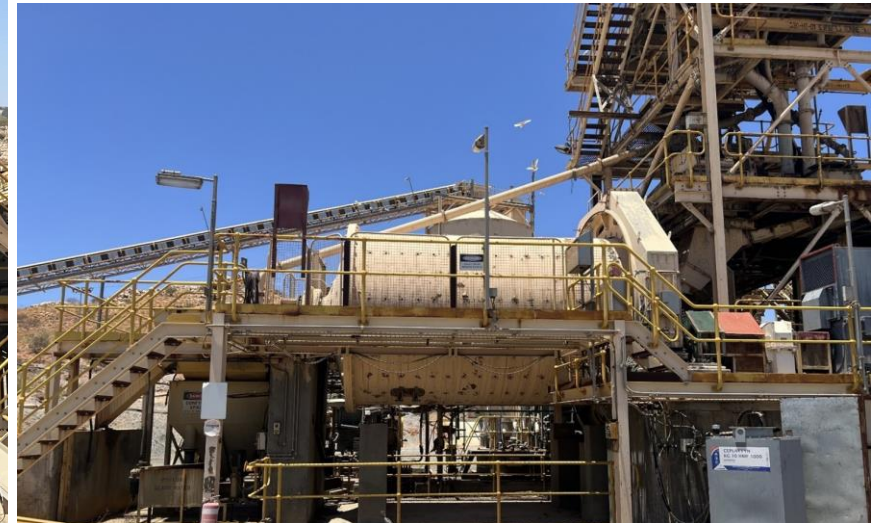
1MW ball mill – liners and lifters ordered
